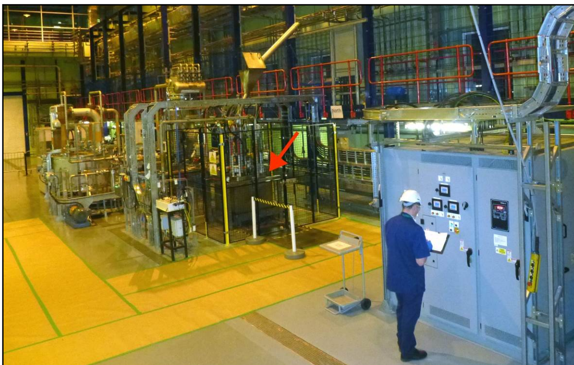
Fig. 6. GeoMelt ICV System at NNL Central Laboratory Active Rig Hall.
